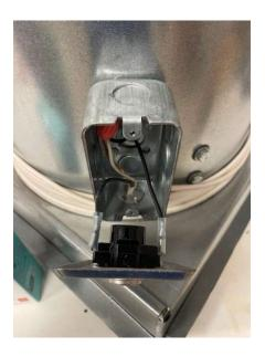
3. **Take Note of Wiring**: Take a moment to observe how the wires are connected to the old switch. There will be two wires connected to the thermostat: a black (hot) wire coming from the Romex (electrical circuit), and a black wire going to the fan. Note which wires are connected to each, as you'll need to reconnect them appropriately to the new switch.
