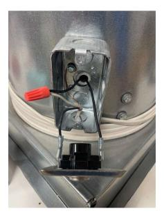
4. **Disconnect Wires**: Remove the wires from the thermostat and cut-off the connectors.
